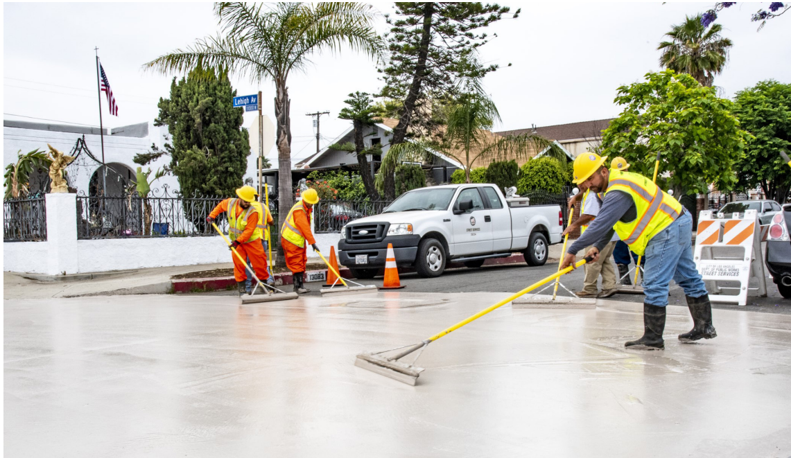
Cool Pavement Work Photo: Los Angeles Bureau of Street Services
