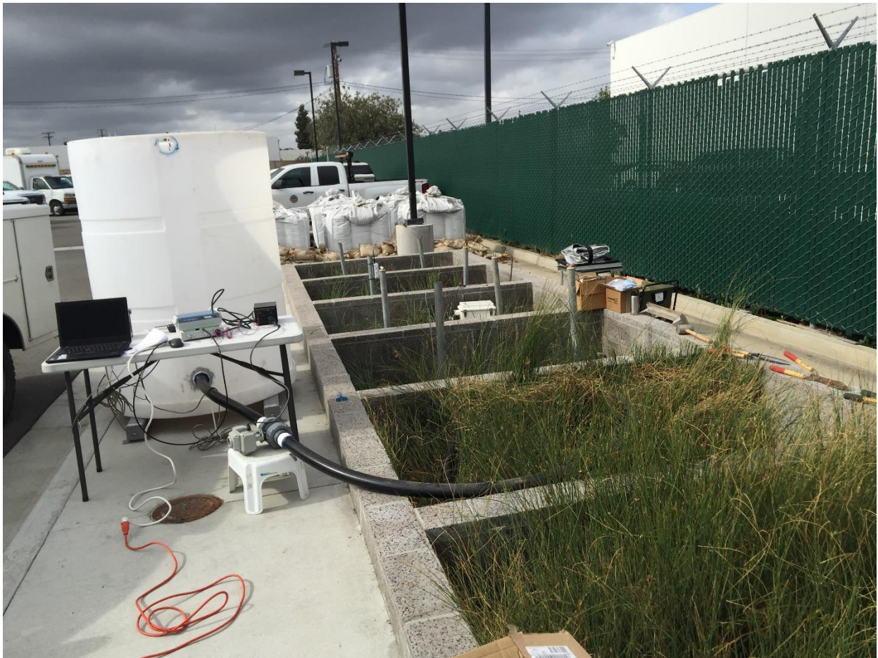
Figure 12: The experimental setup consisted of a 500-gallon tank with a trash pump to ensure homogenous concentration of the influent. The control valve is pictured on the white stool.
