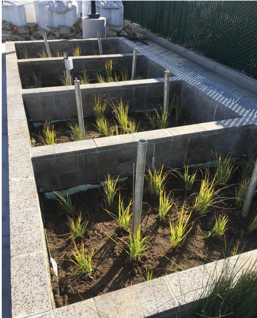
Figure 12: The cells were vegetated with Carex spissa and contained six spray heads for irrigation. In addition to infrequent rains received since completion of construction and planting, the biofilter cells were mainly irrigated with tap water to support plant growth. Biweekly weeding was implemented to maintain a monoculture plant species in these four biofilter cells.
