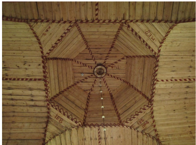
The inner ceiling in the church at Petäjävesi
