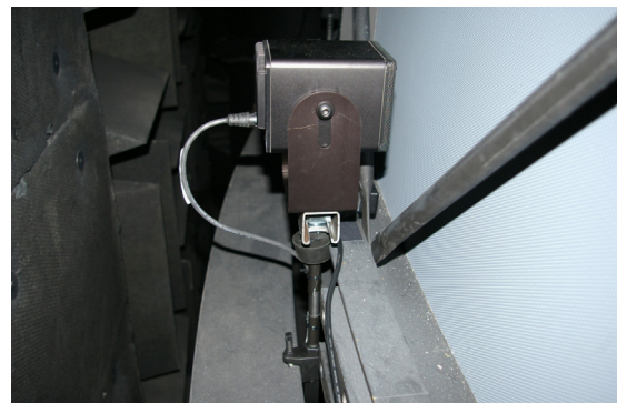
Fig. 11. Meyer MM4XP loudspeaker on custom mount. Left side of image shows sound absorption materials and right side shows the back of the projection screen.
