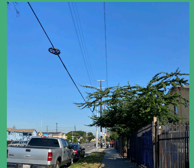
Figure 4. Overhead power lines
