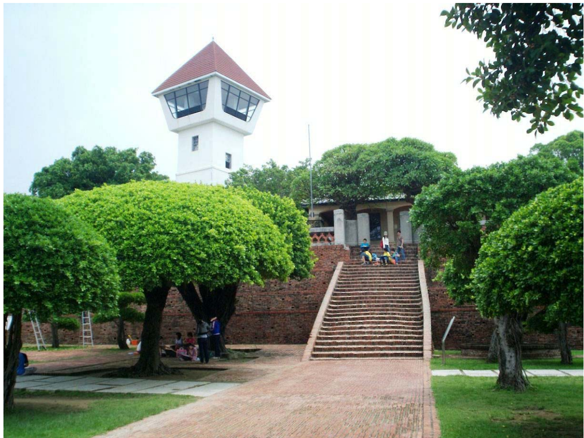
Figure 23. Casteel Zeelandia, which later became the Zheng family's headquarters on Taiwan. Today, only the foundations remain of this once-impressive defensive network. On top of it, the Qing maintained a garrison until the late nineteenth century, just before Taiwan was ceded to Japan. The grounds of the fortress then became converted into an observation deck and a dormitory for customs officers.
