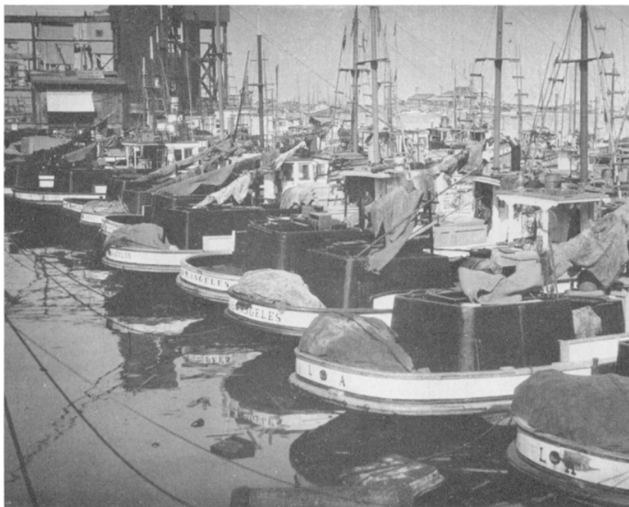
FIGURE 4. Albacore live-bait vessels. Note bait tank and trolling poles. Photo by G. R. Chute, 1927.
