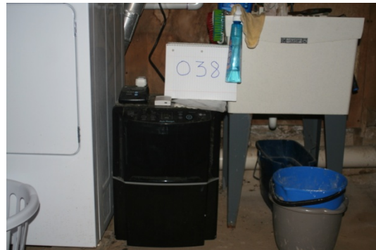
Figure 11-5 Dehumidifier with clothes dryer
