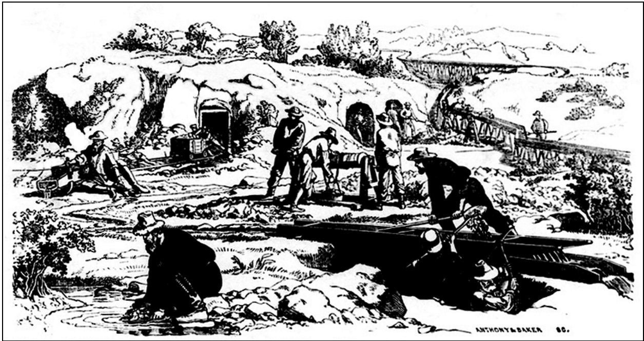
Figure 2.3. “Traditional” placer mining techniques including sluicing, tommying, cradling, panning, drifting, tunneling, fluming, and shafting. Source: “How the California Mines are Worked,” The Wild West , December 1, 1854, 1.
