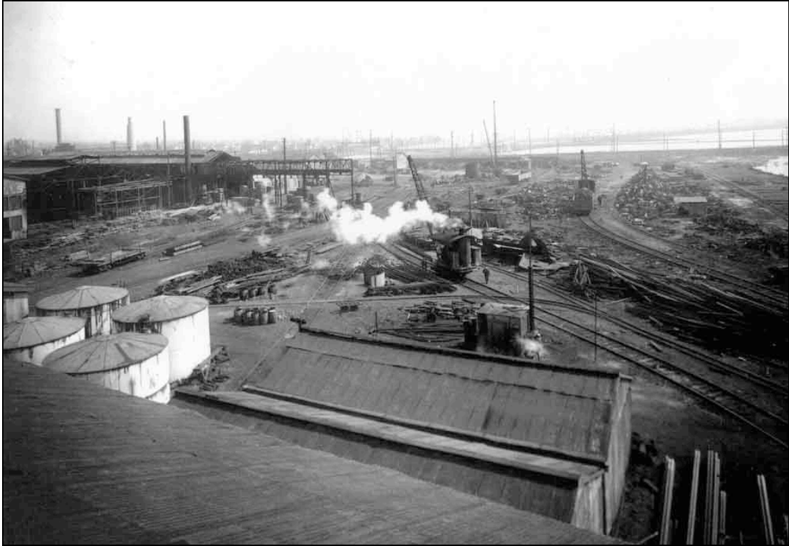
Figure 5.13. Judson Manufacturing Company expanded southward using slag as bayfill. Source: Emeryville Historical Society.
