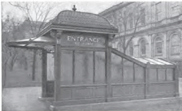
One of the 111 Kiosks for Rapid Transit Subway, New York Heins & LaFarge, Architects. Wm. Barclay Parsons, Chief Engineer Executed by Hecla Iron Works
