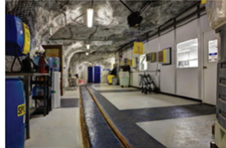
FIGURE 12: A photograph of the TCR used for electroforming on the 4850' level at SURF.
