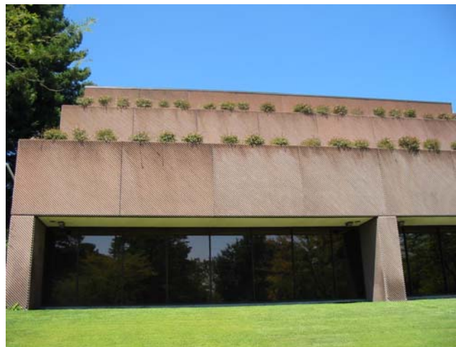
Figure 2.3. Santa Rosa Federal Building
