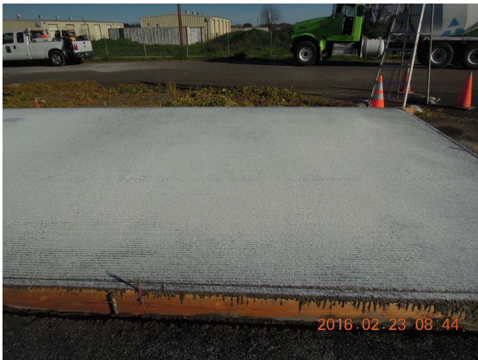
Figure A.50: Section with curing compound already applied.
