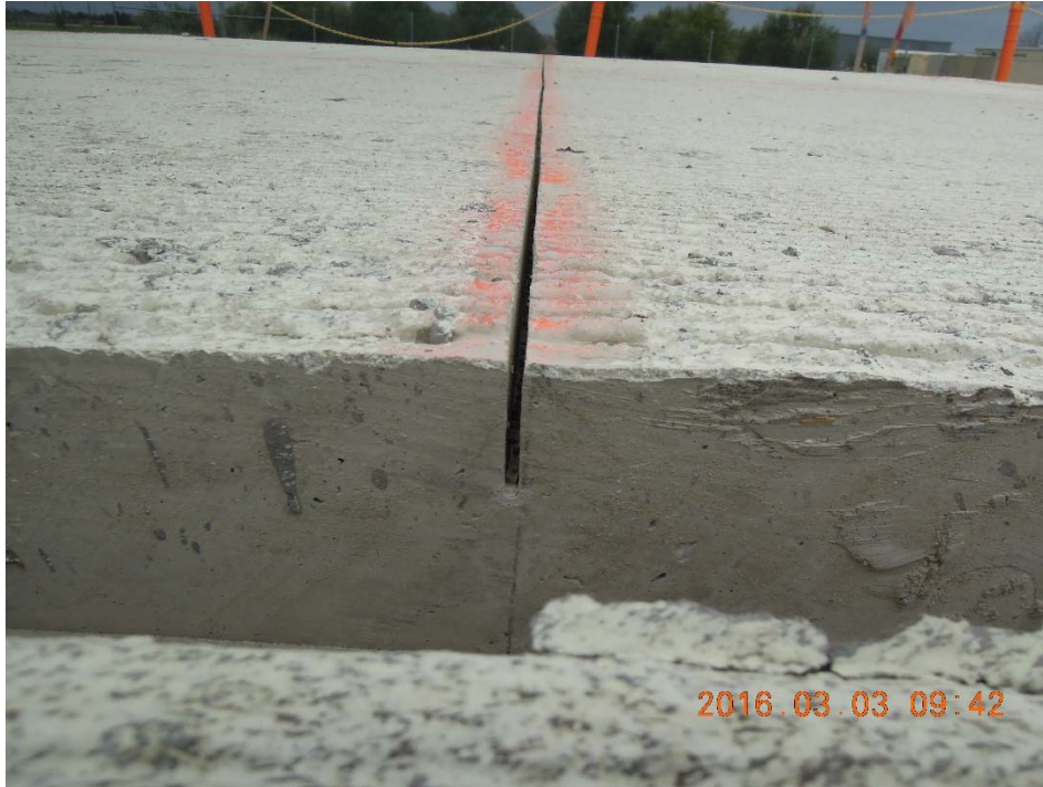
Figure A.105: Saw cut to 1/3 of PCC depth.
