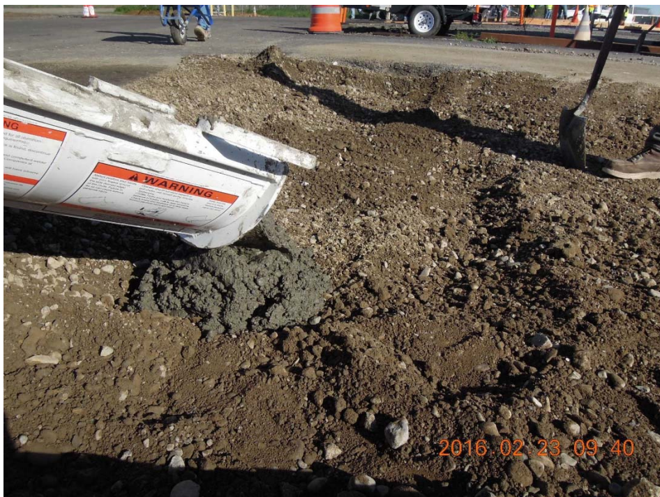
Figure A.52: Disposal of leftover concrete.
