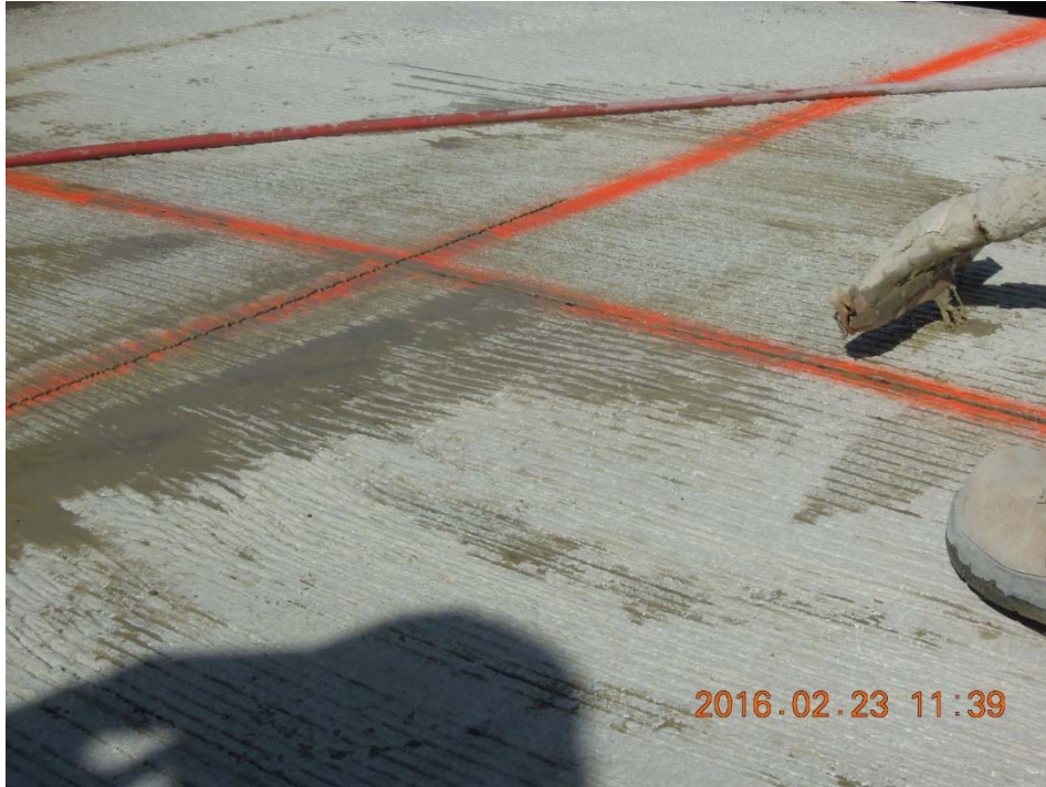
Figure A.75: Vacuum cleaning after saw-cutting.
