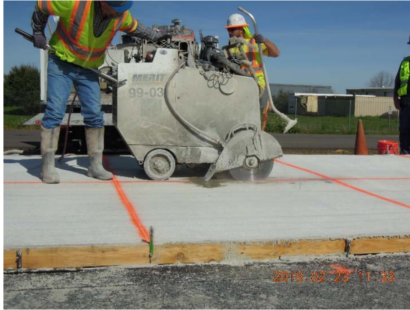
Figure 4.13: Saw-cutting operation.
