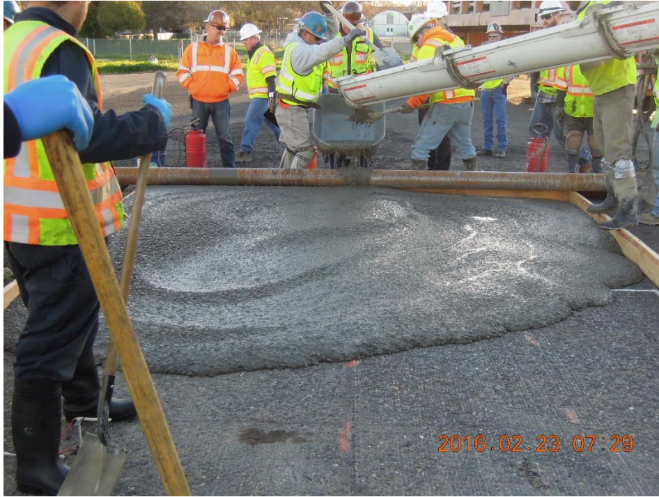
Figure A.35: Sampling of concrete for QC/QA.
