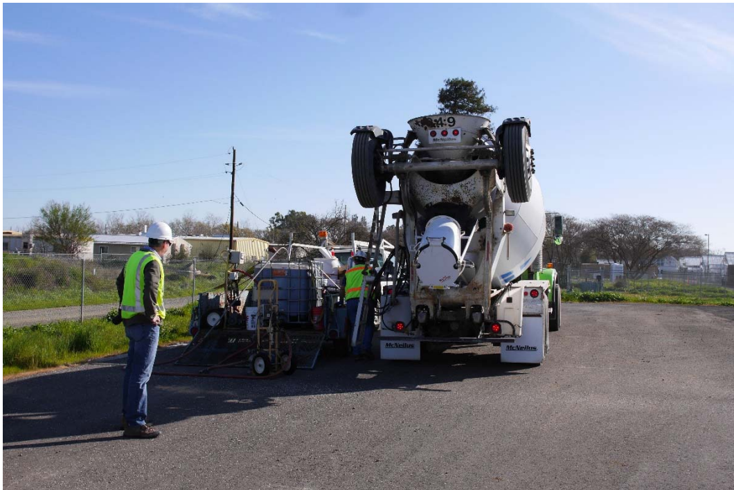
Figure A.96: Accelerator dosing into the ready-mix truck.
