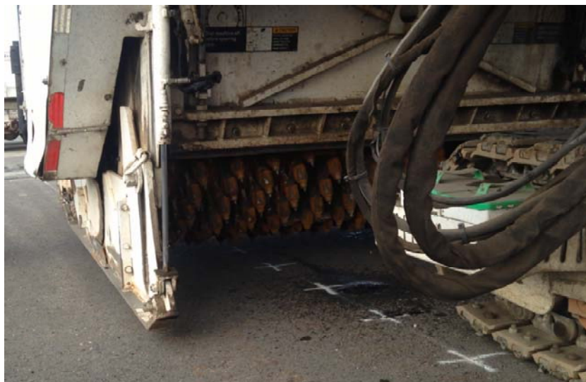
Figure 4.1: Milling machine with micromilling teeth spacing.
