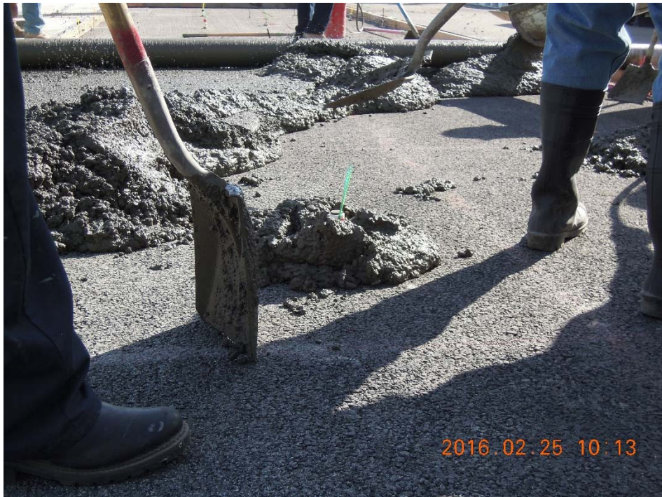
Figure A.86: Pouring concrete around instrumentation.
