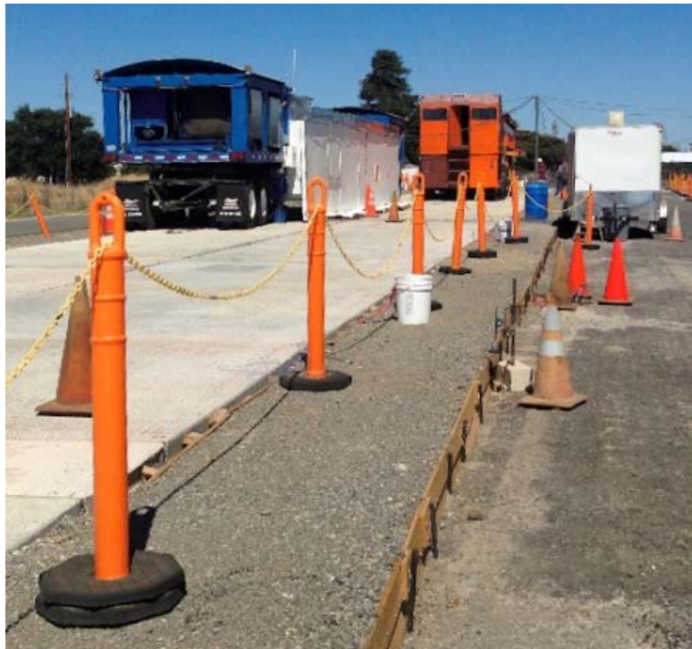
Figure 4.23: Granular shoulders of the test track.
