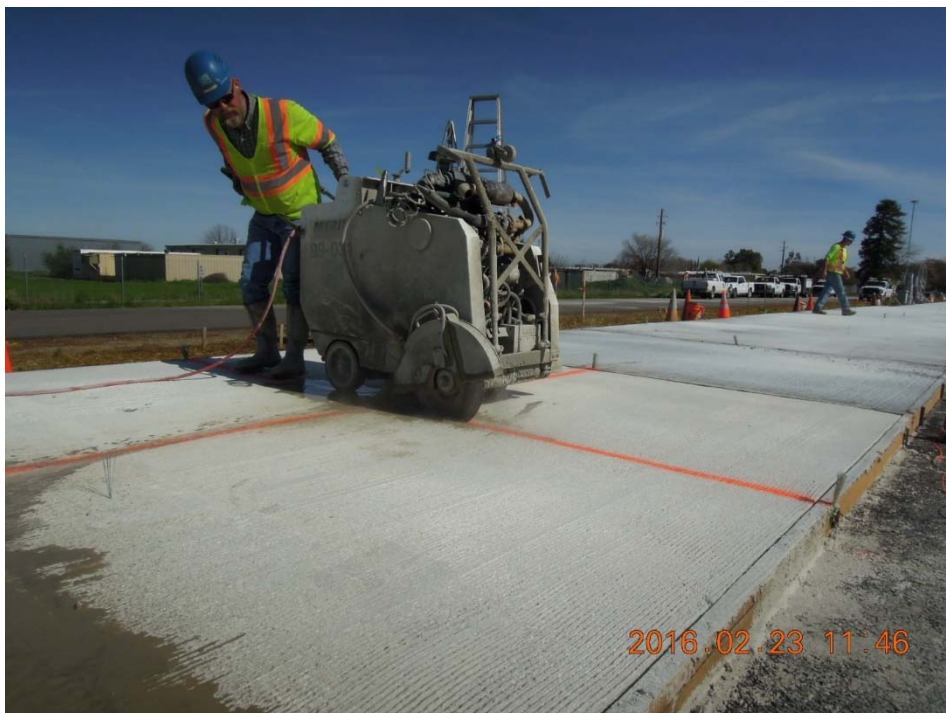
Figure A.76: Saw-cutting transverse joints.
