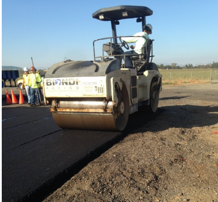
Figure A.5: Roller compaction of the edge of the HMA layer.
