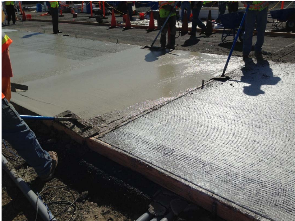
Figure A.66: Section edge finishing.
