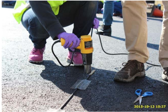
Strain gage on top of HMA, before FAM protection
