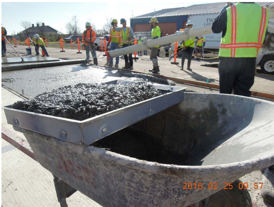
Figure A.82: Wet sieving of concrete for preparing the unrestrained shrinkage beams.
