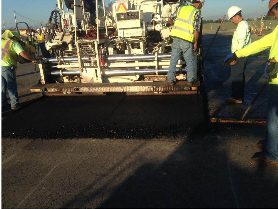
Figure A.3: Hot mix asphalt (HMA) paving.
