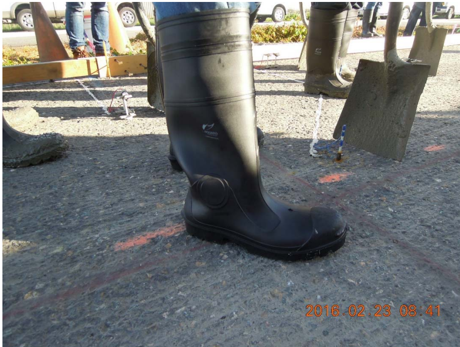
Figure A.49: Protecting the instrumentation before concrete pouring.
