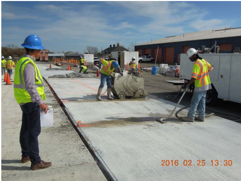
Figure A.88: Saw-cutting and vacuum cleaning.
