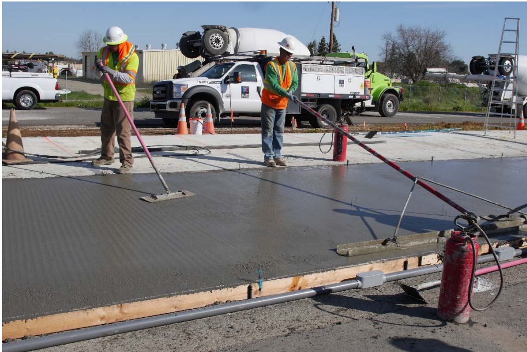
Figure A.98: Bull-float finishing.
