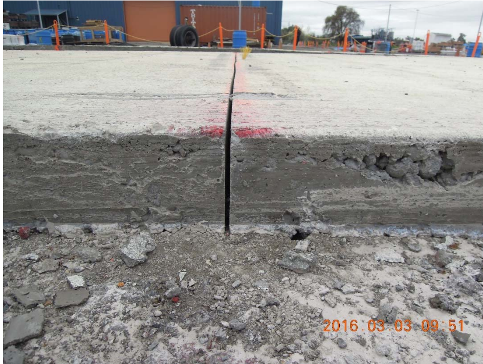
Figure A.107: Full-depth cut for separating sections.
