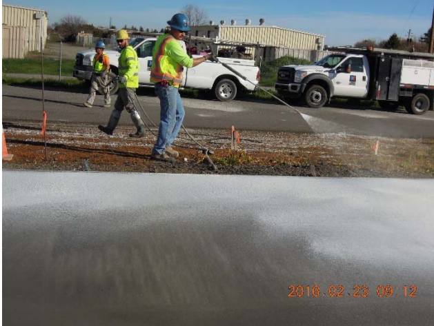
Manual spraying of curing compound
