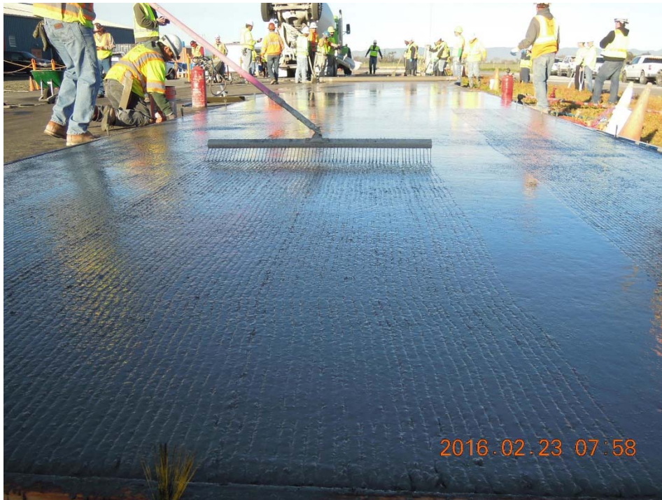
Figure A.43: Metal rake tining of the concrete surface.
