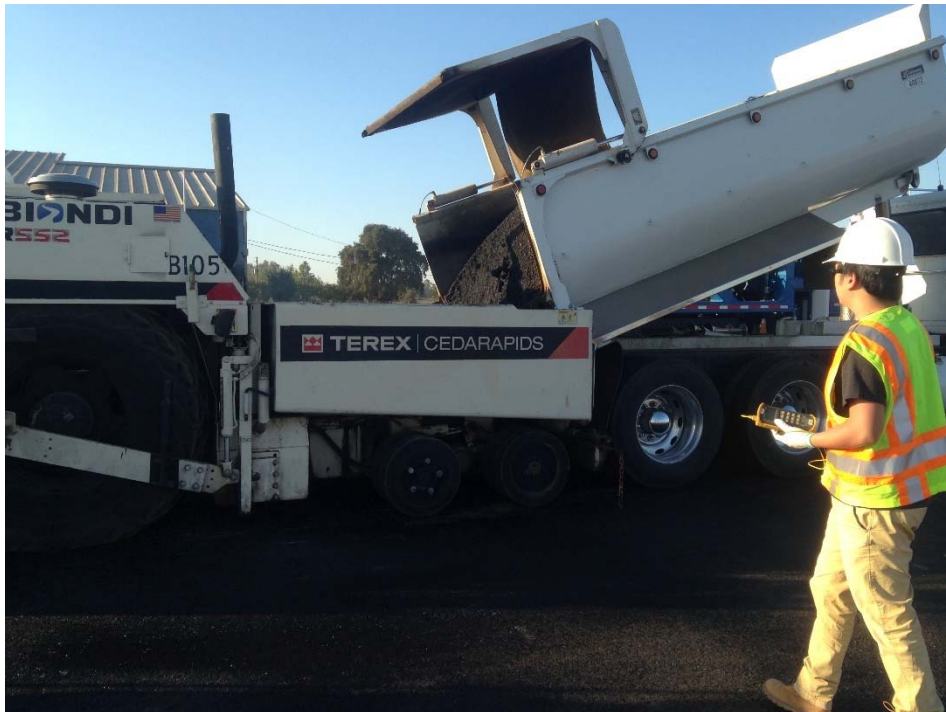
Figure A.4: HMA being dumped into the asphalt paver.
