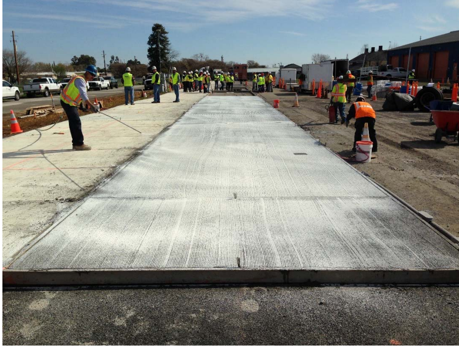
Figure A.91: Manual application of curing compound.
