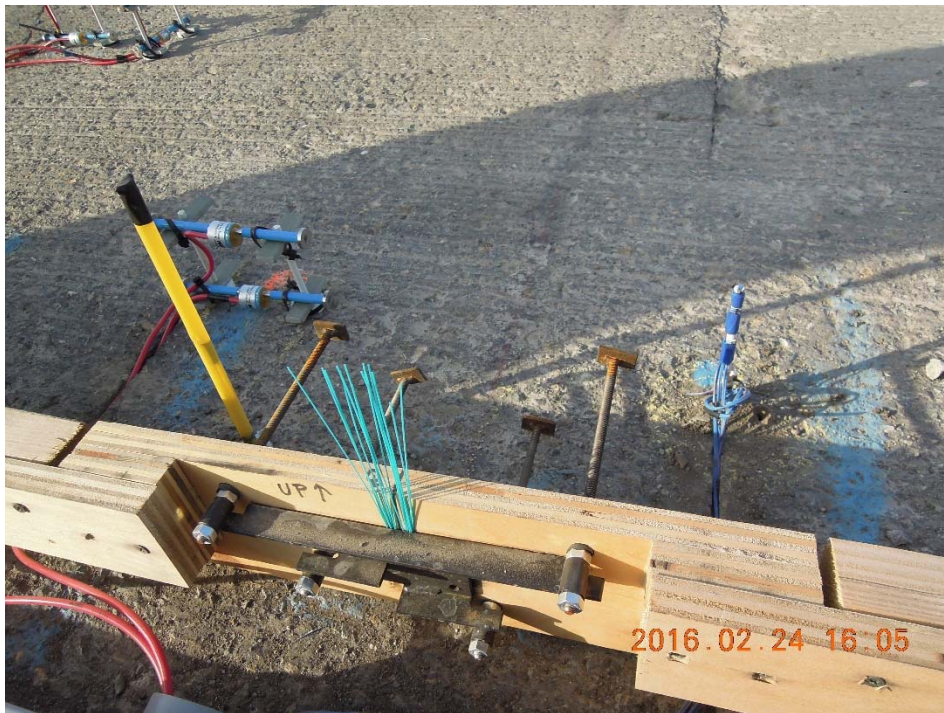
Figure A.24: From left to right: static strain gages, IOMD rod, anchoring rods for the JDMD targets, and thermocouples attached to a fiberglass rod.
