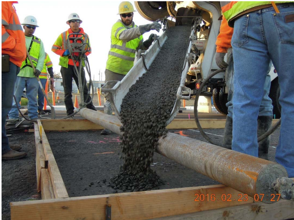
Figure A.34: Pouring concrete at the beginning of the section.
