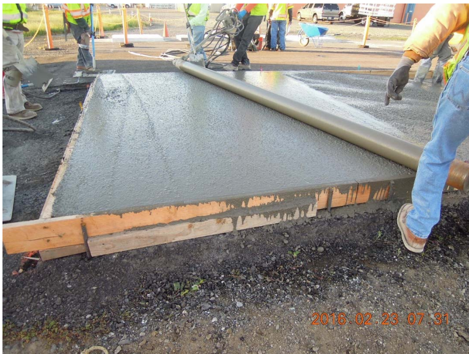
Figure A.36: Hand-rolling screed for concrete consolidation.
