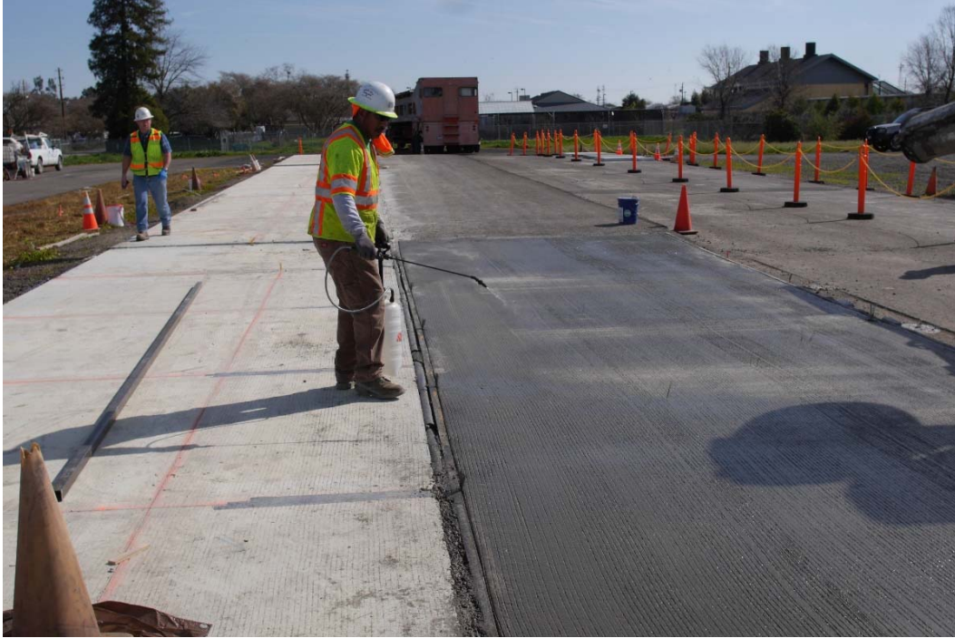
Figure A.99: Manual application of shrinkage-reducing admixture.
