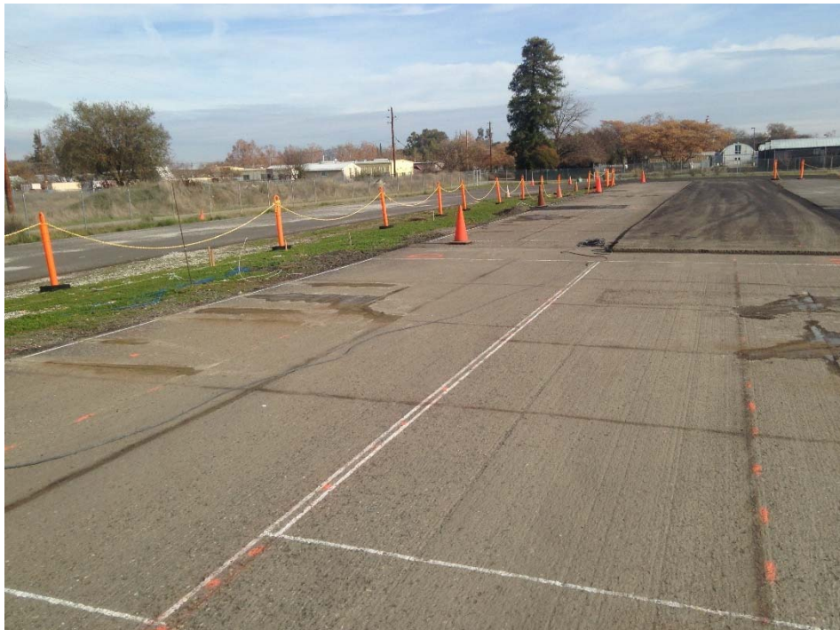
Figure A.12: Micromilled old HMA surface.
