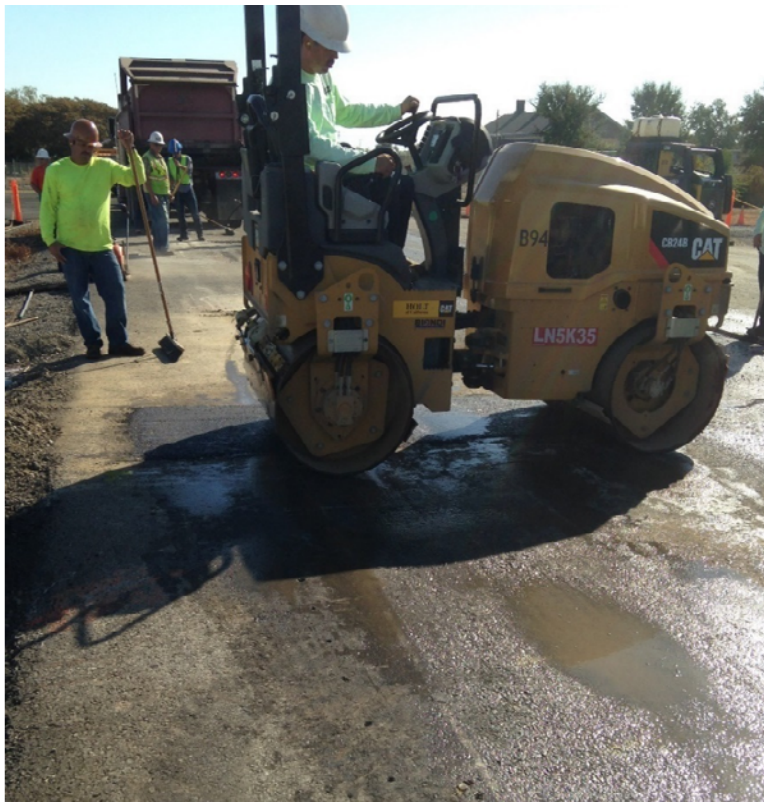
Figure A.8: Compaction of patch on distressed area of the test track.
