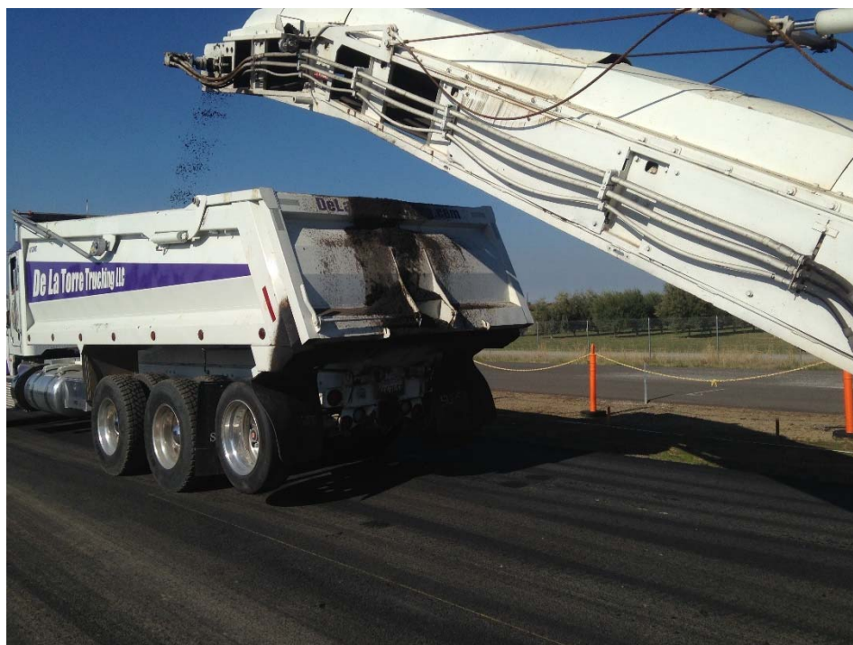
Figure A.10: Disposal of milled material.
