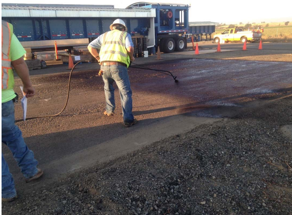
Figure A.2: Application of prime coat on top of FDR layer.
