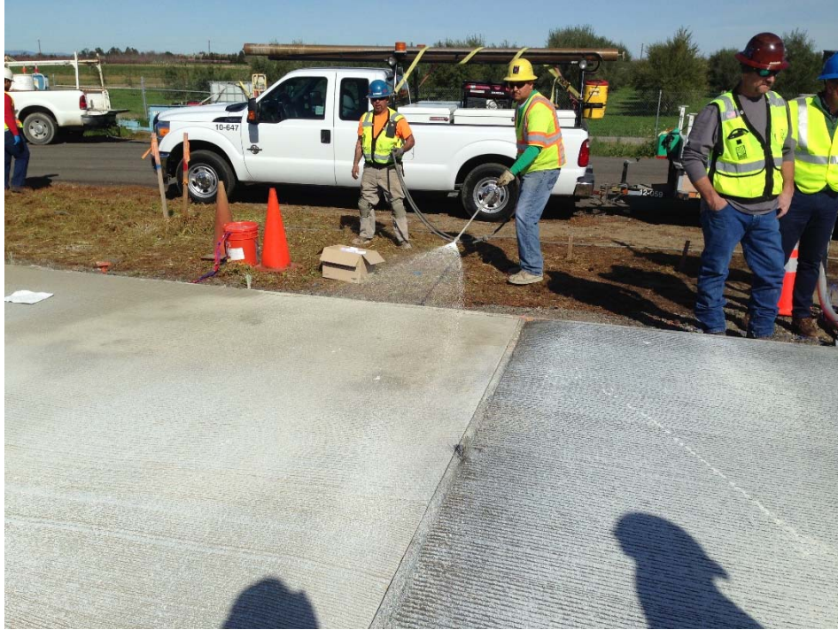
Figure A.63: Curing compound application.
