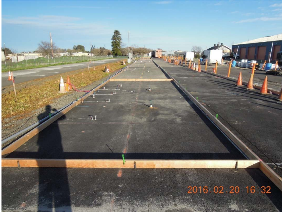
Figure A.15: Lane 1 ready to be paved.
