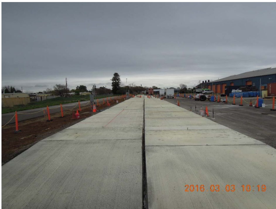
Figure A.116: Longitudinal view of the test track.
