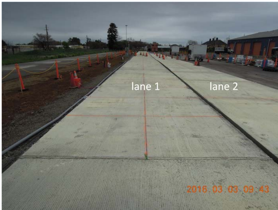
Figure 4.17: Full-scale test-track after overlay construction.
