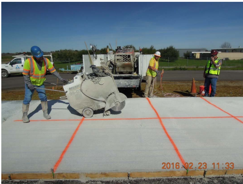
Figure A.74: Saw-cutting.
