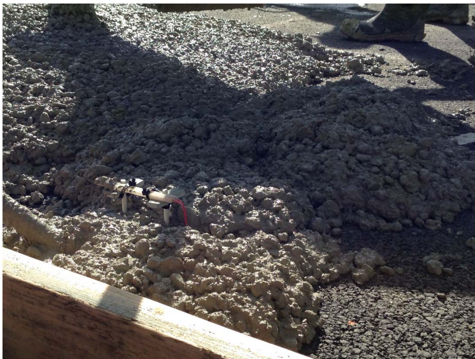
Figure A.56: Pouring concrete around instruments.
