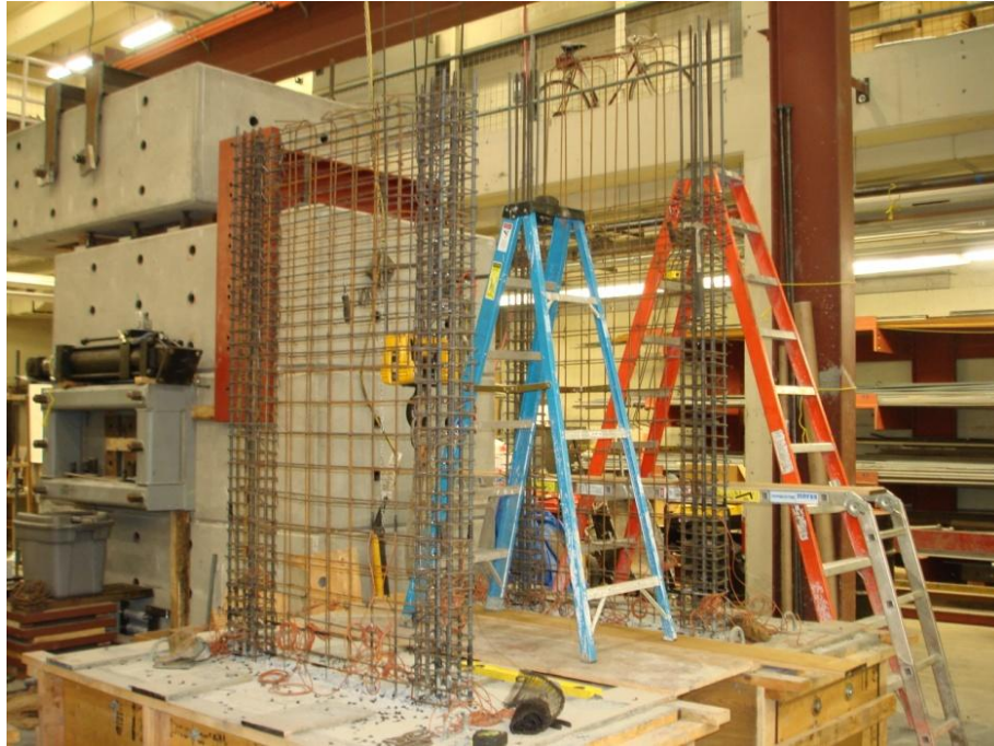
Figure 5-11 Fabricating boundary transverse and web horizontal reinforcement
