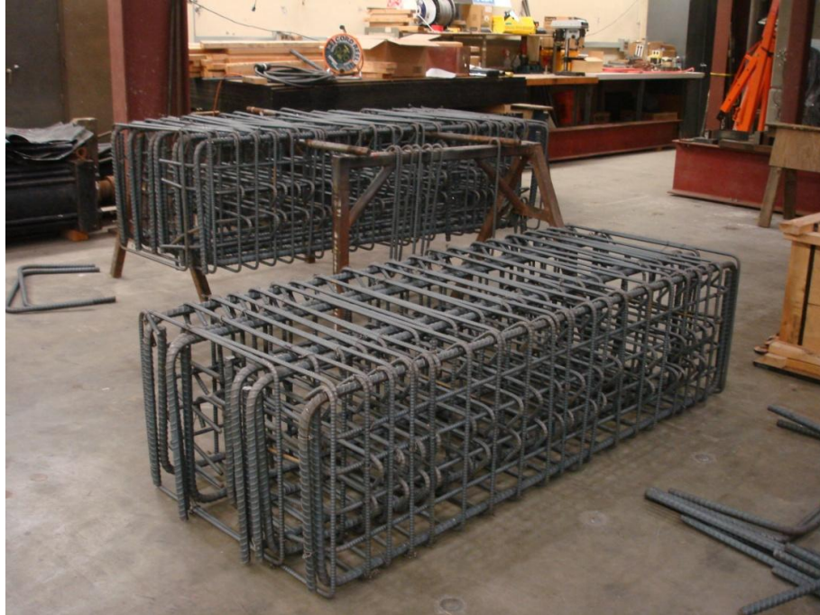
Figure 5-7 Making reinforcement cages for the foundation blocks
