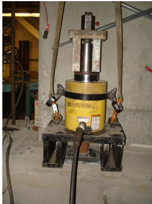
Figure 4-5 Post-tensioning a typical anchor bar
