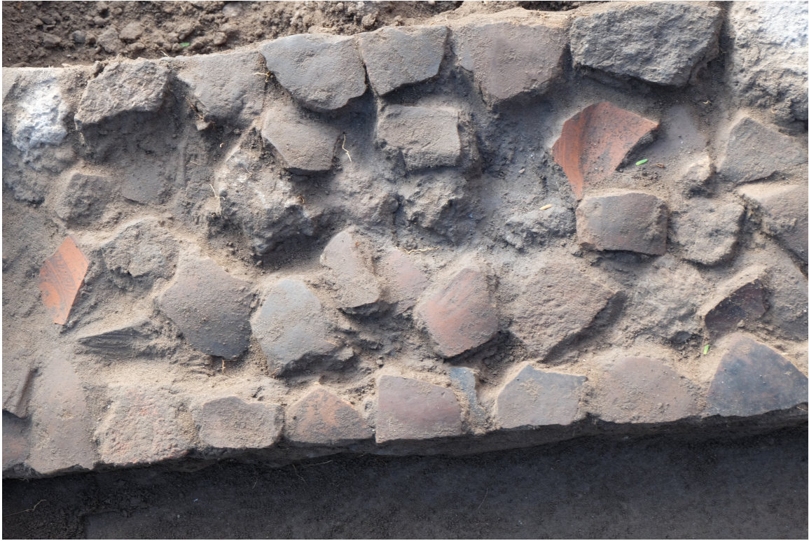
Figure 6.2. Ceramic-lining of wall foundation.
