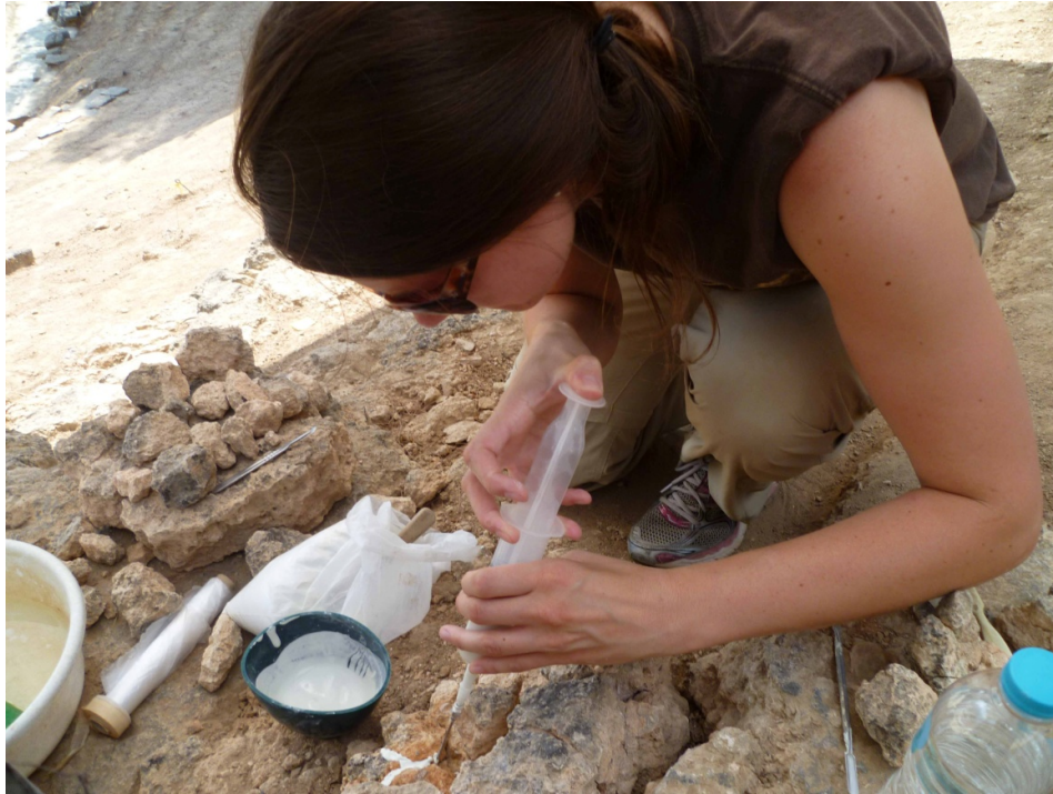
Fig. 8: Photo of author injecting grout into fissures in weathered sandstone seats in the field at the Theatre of Demetrias, Volos, Magnisia, Greece (Courtesy of Hara Topa, 2012)
