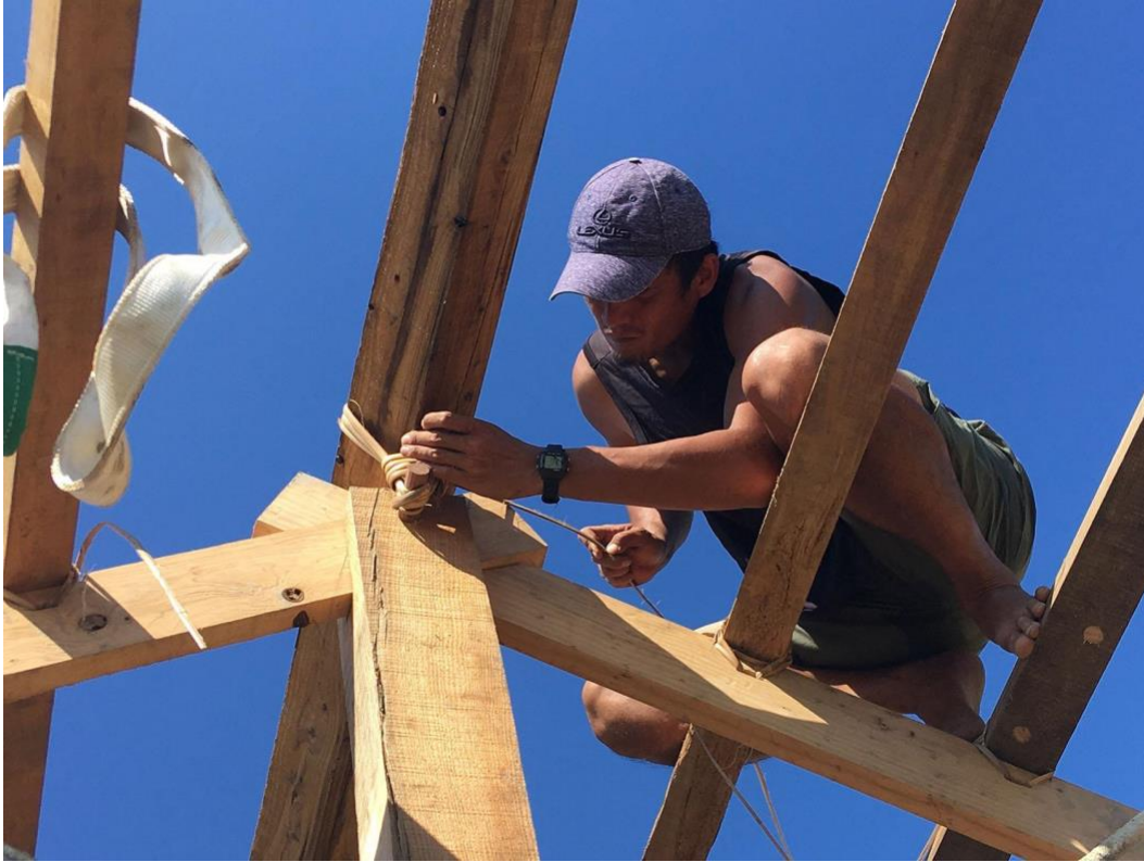
Figure 2. Akac Orat using rattan for structural binding on a traditional Amis house, Madawdaw, Taitung County, Taiwan, 2020. Photograph courtesy of Hau En Tsai
