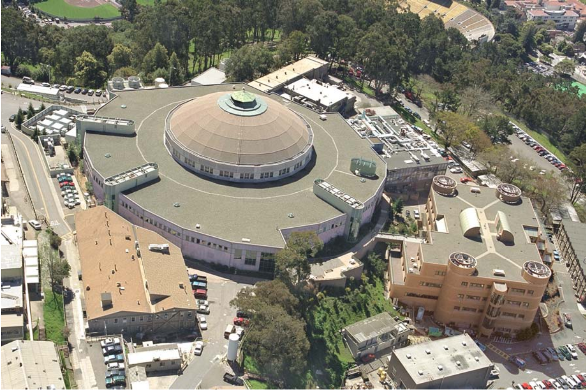
Figure 1 (XBD9904-00696.jpg). Aerial view of the ALS at the Ernest Orlando Lawrence Berkeley National Laboratory. The ALS building consists of an older central portion (under the dome) and the newer annular structure around it. The dome was retained from the historic 84-Inch Cyclotron, whose large size prompted Lawrence to establish a new laboratory on the hillside above the University of California, Berkeley, campus during the World War II years. (Lawrence Berkeley National Laboratory Photographic and Digital Imaging Services)
