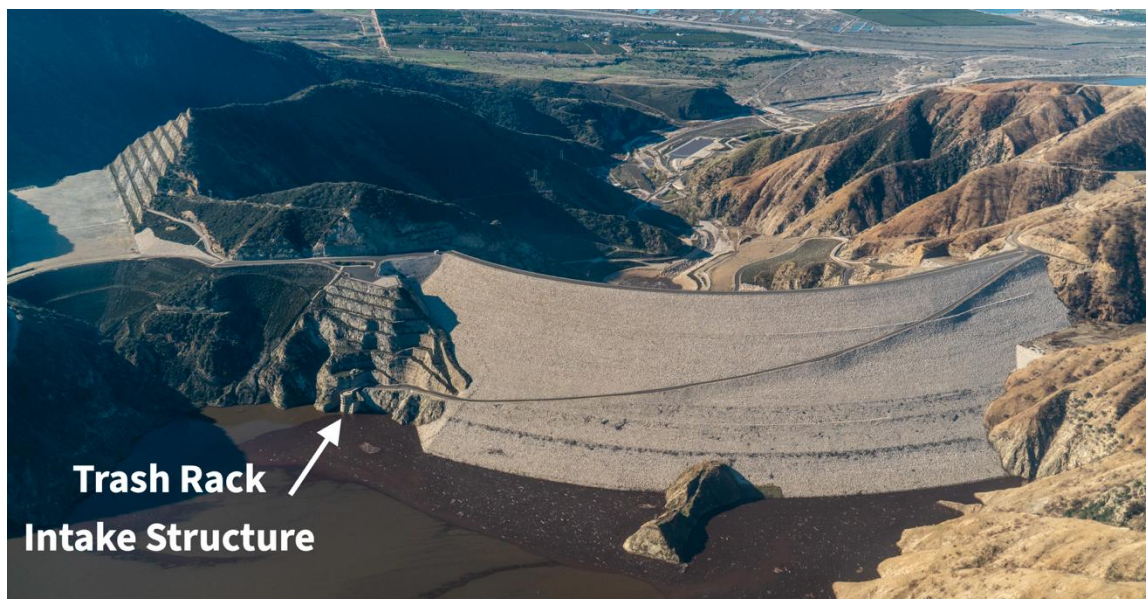
Figure 3-2. Aerial photograph of Seven Oaks Dam and Reservoir. (Credit: Orange County Water District and EcoFlight.)
