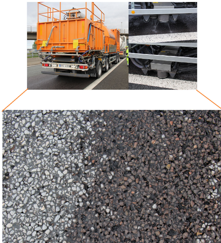
Figure 5.3: Vägren truck high-pressure cleaning equipment used for OGFC cleaning in Sweden. (Source: Ahmed 2015)
