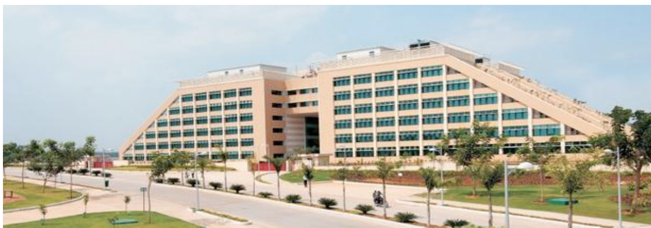
FIGURE 13: The SDB-1 building at Infosys, Pocharam. A comparison between the two wings—one with a conventional VAV system and the other with a radiant cooling system—reveals the benefits of a radiant system. (Photo: Infosys Green Initiatives Team)
