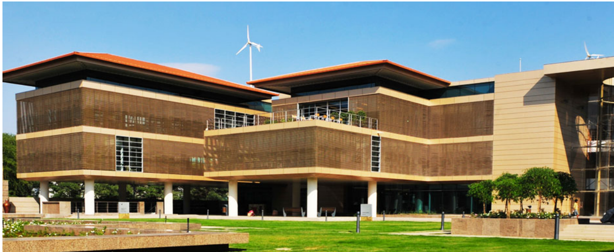
FIGURE 33: Use of louvers and the mass of the building's blocks to shade the large glazed areas at Suzlon One Earth, Pune. The glazing has low-E glass, there is extensive over-deck insulation provided, and the height of the buildings is kept deliberately low--all factors that substantially reduce the envelope heat gain. (Photos: Synefra 13 )
