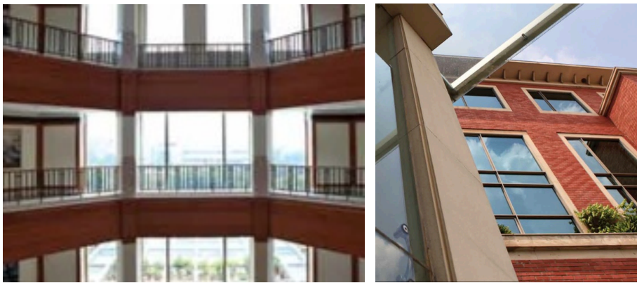
FIGURE 27: ITC Green Center, Gurgaon, showing the daylighted atrium and façade with low-E windows. (Photos: ITC) 22
