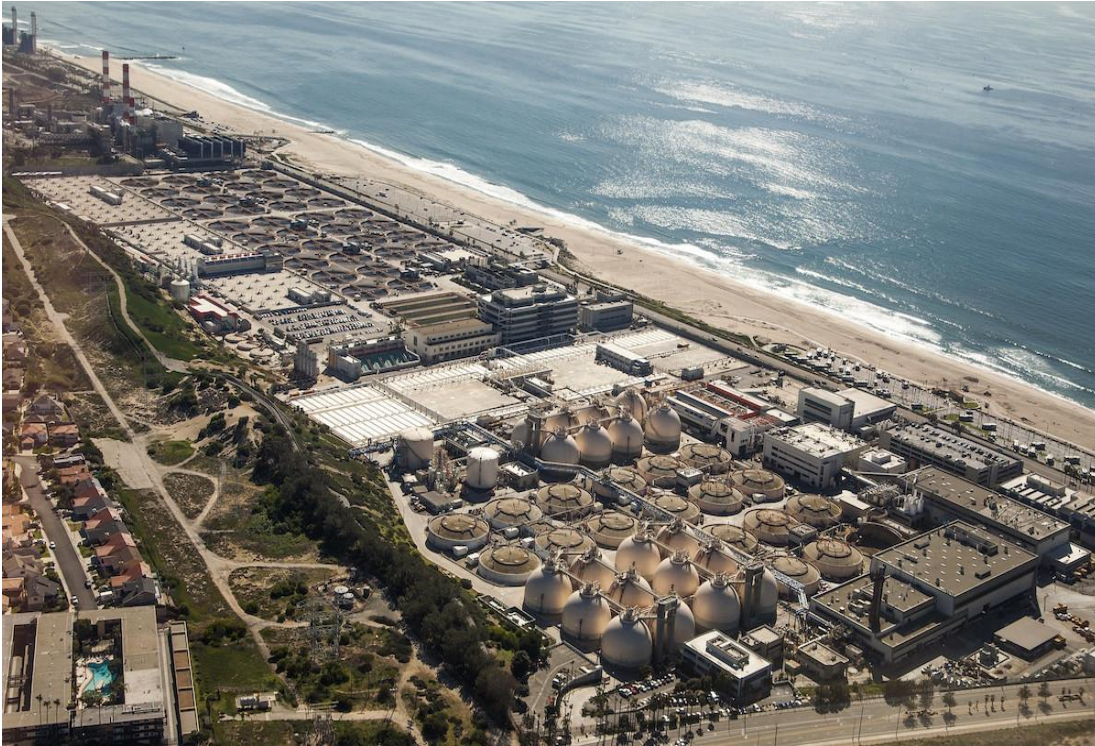
Figure 2. Hyperion Water Reclamation Plant, LA Sanitation & Environment - City of Los Angeles.
