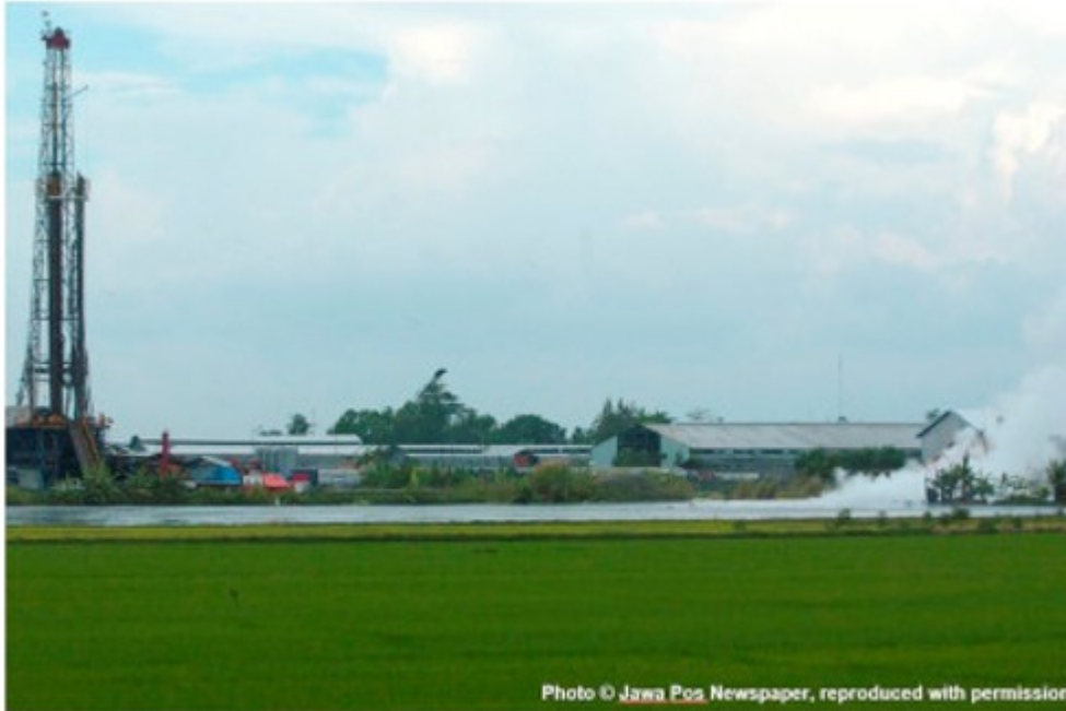
Fig. 7. Photo of the TMMJ drill rig and BJP-1 location and the first documented Lusi eruption site approximately 100 m from the well (“40ft SW of flare pit”). Exact time of the photograph is not documented, but is within the first 3 days of the Lusi eruption, as the drill pipe is clearly still visible in the racks on the rig tower, and daily drilling reports note that this was removed before sunrise on the 2nd of June. Photo from Guslan Gumilang/Jawa Pos, with permission.
