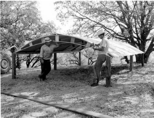
Marshall Slater and Richard Rainoldi check newly-completed sheep shelter utilizing thin plastic roofing material, November 1966
