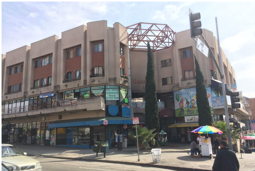
Figure 6.7: Grande Mall, on the ground floor, is the retail anchor of this mixed use building of 1990s vintage. Photo by author, 2014.
