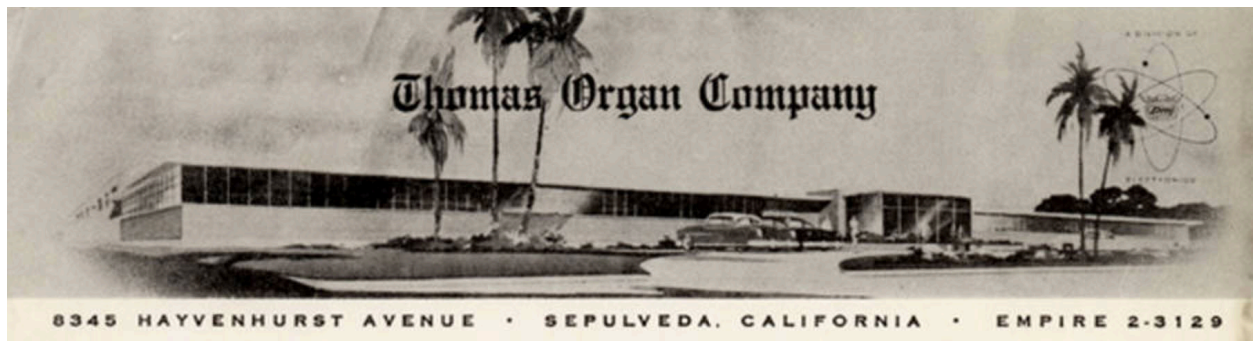
Figure 2.19: The Thomas Organ Company factory pictured on company letterhead, circa 1950s. The building would be repurposed as the Valley Indoor Swap Meet in 1983.
