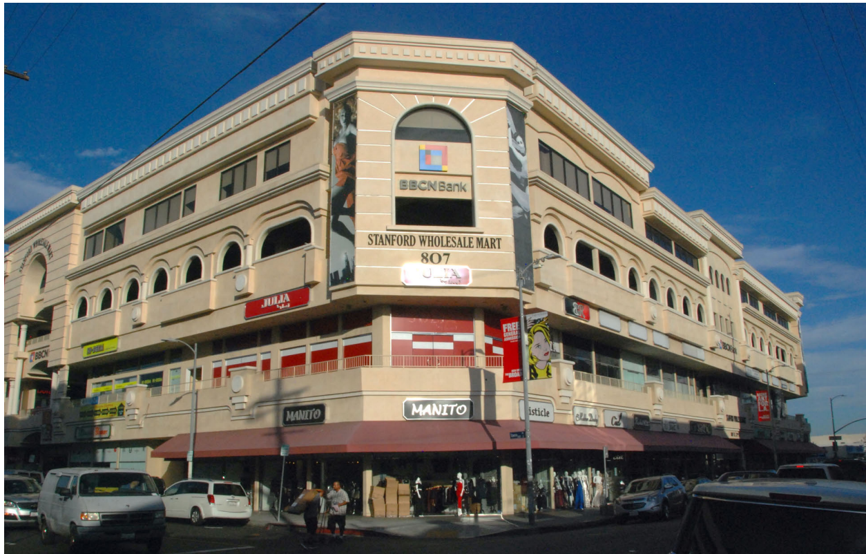
Figure 3.25: The Stanford Wholesale Mart at the intersection of 12 th Street and Towne Avenue in the Los Angeles Fashion District is one of several massive “marts” which house hundreds of garment wholesalers. Within each firm’s showroom, retailers may purchase bulk quantities of apparel for sale in their stores. The BBCN Bank sign (near the top of the building) signals the presence of at least six different Koreatown-based banks, which operate branches in the District and cater to Korean-owned wholesale and garment contracting firms. Photo by author, 2015.
