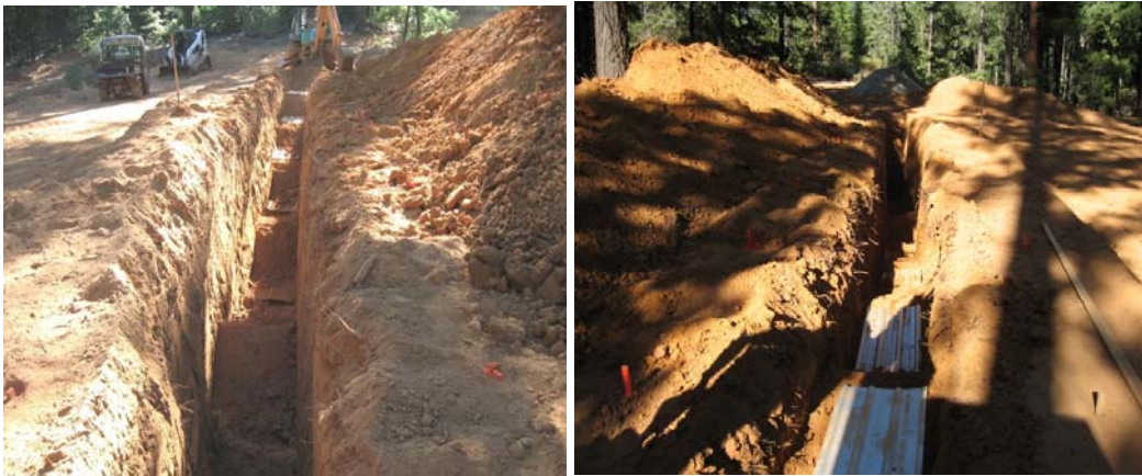
Figure 5.2. Tin roofing Sheets buried at different Depths at Forest Lodge
