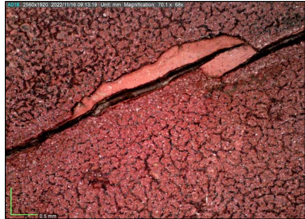
Figure 21: Photomicrograph of multiple red layers visible along a crack.
