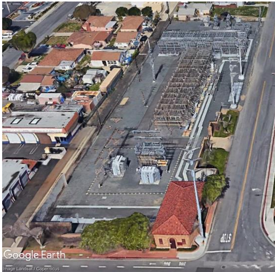
Figure 4.2 – View of Ocean View Substation from Google Earth.
