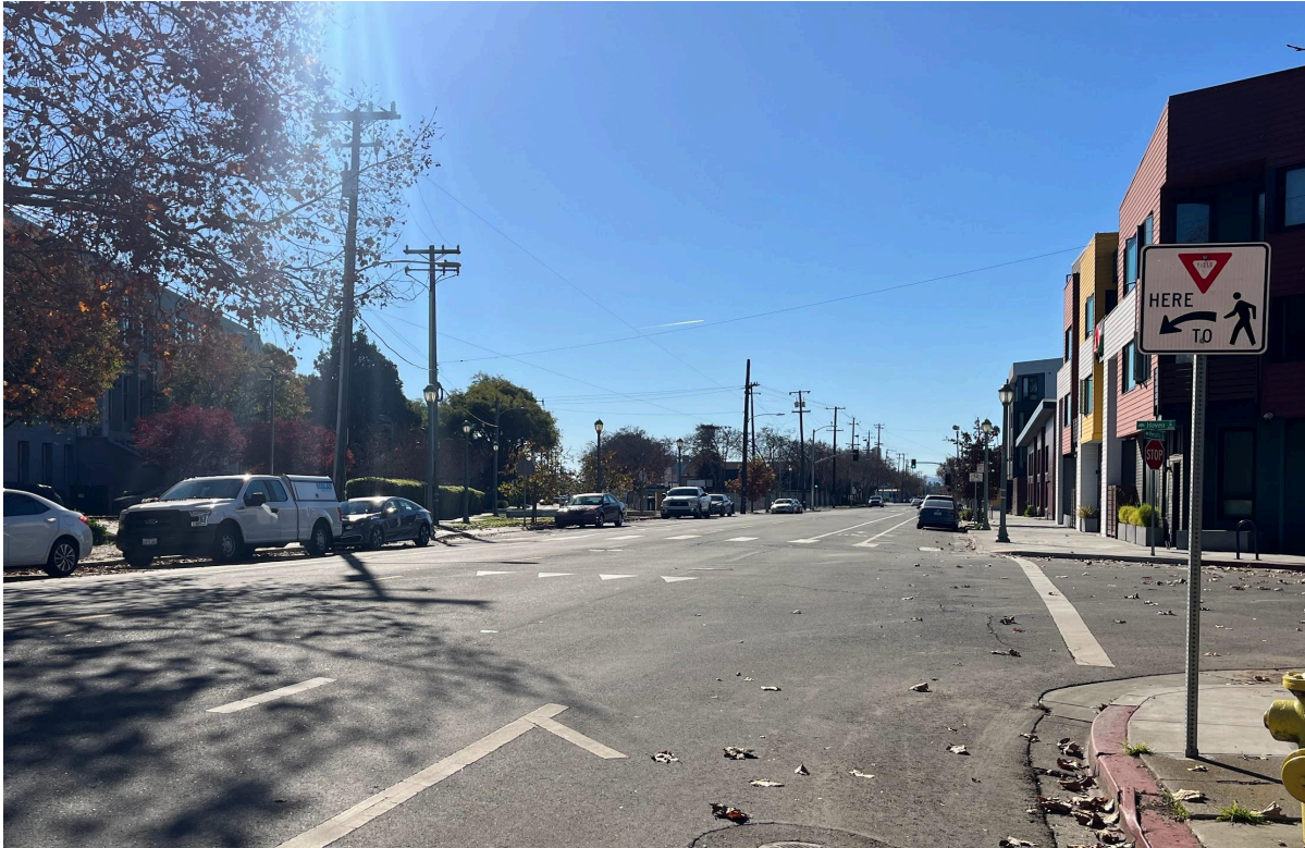
Image: Bicycle Lane, Pedestrian Signage, and High-Visibility Crosswalk at Peralta St and Haven St, 2024 | Photo Credit: Natalie Martinez
