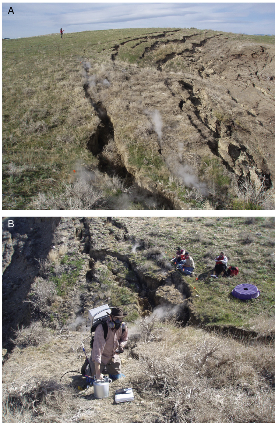
Fig. 2. A) Photograph of arcuate fractures in developing part of Ankney fire. The most intense part of the fire, generally towards the lower right corner of the picture, has not yet undermined this area, but subsidence related to the fire-related removal of the coal has begun. B) Photograph of the Ankney fire. Soil CO 2 flux measurements in foreground; measuring in situ gas composition, and collection of volatile organic gas samples in the background. The most intense part of the fire is to the left of the picture.
