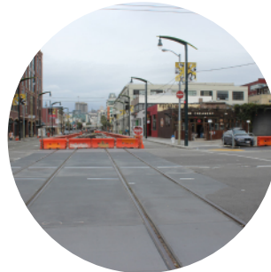
Construction poses another hazard for cyclists moving through the area.
