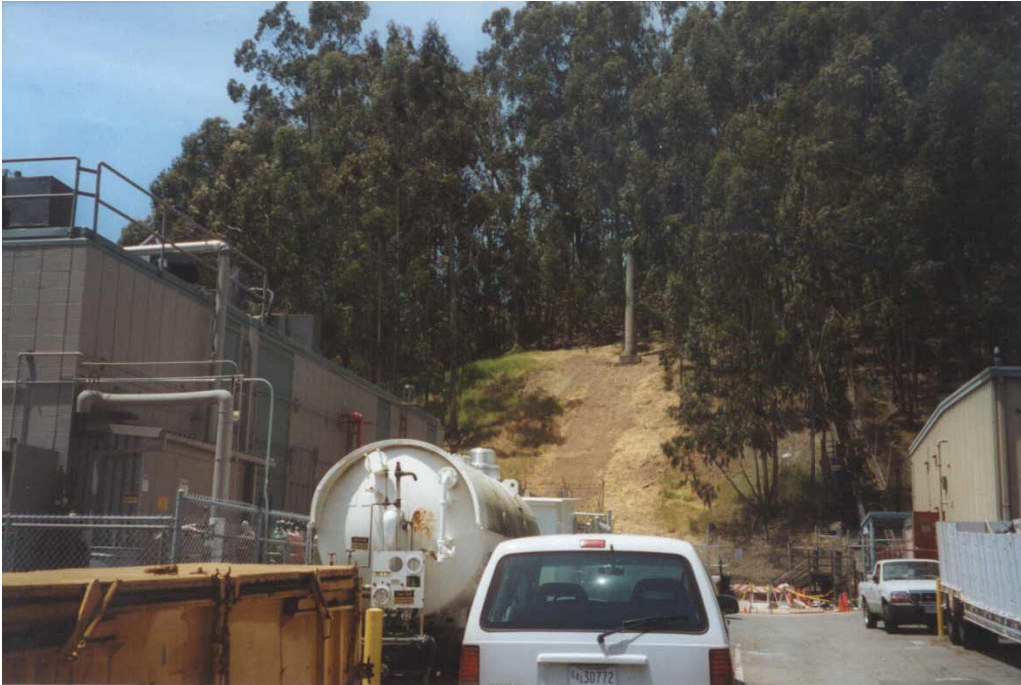
The stack through which airborne tritium is released from the NTLF is located upslope of the facility.
