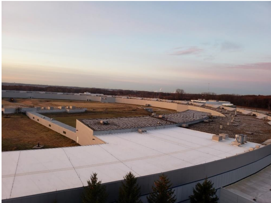
Advanced Photon Source ring, from the balcony of the User Building.
