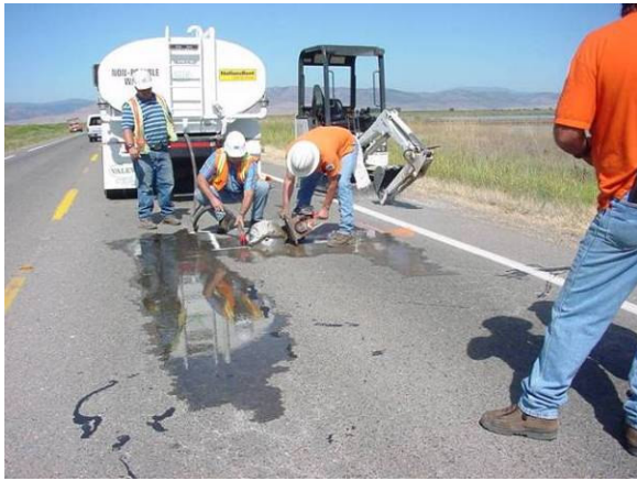
Test pit sawing
