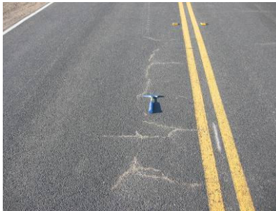
Pumping in new overlay
