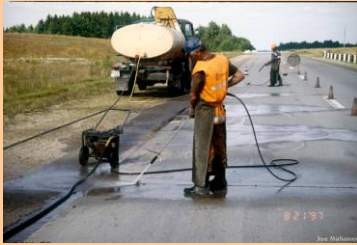
Routine maintenance - crack repair
