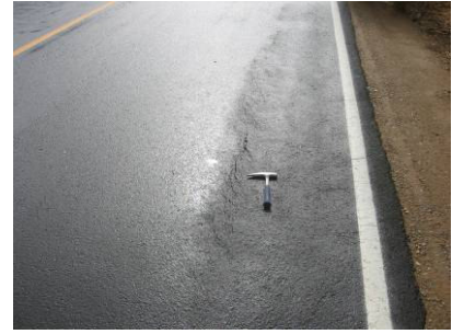
Surface deformation
