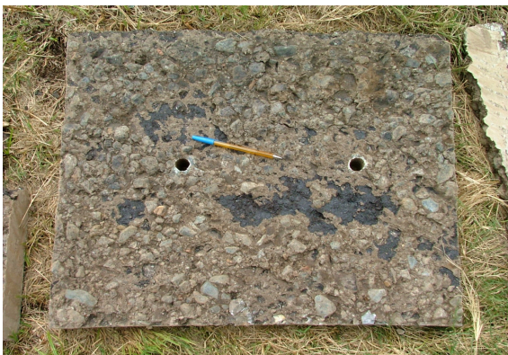
Investigation of slab underside
