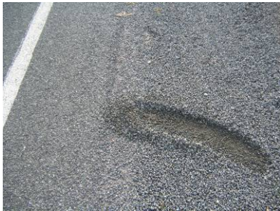
Ravelling from chip seal
