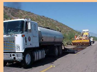
Pavement preservation - chip seal
