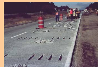
Preventive maintenance - dowel bar retrofit
