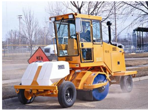
Brooming of excess chip seal stone
