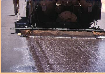
Slurry seal
