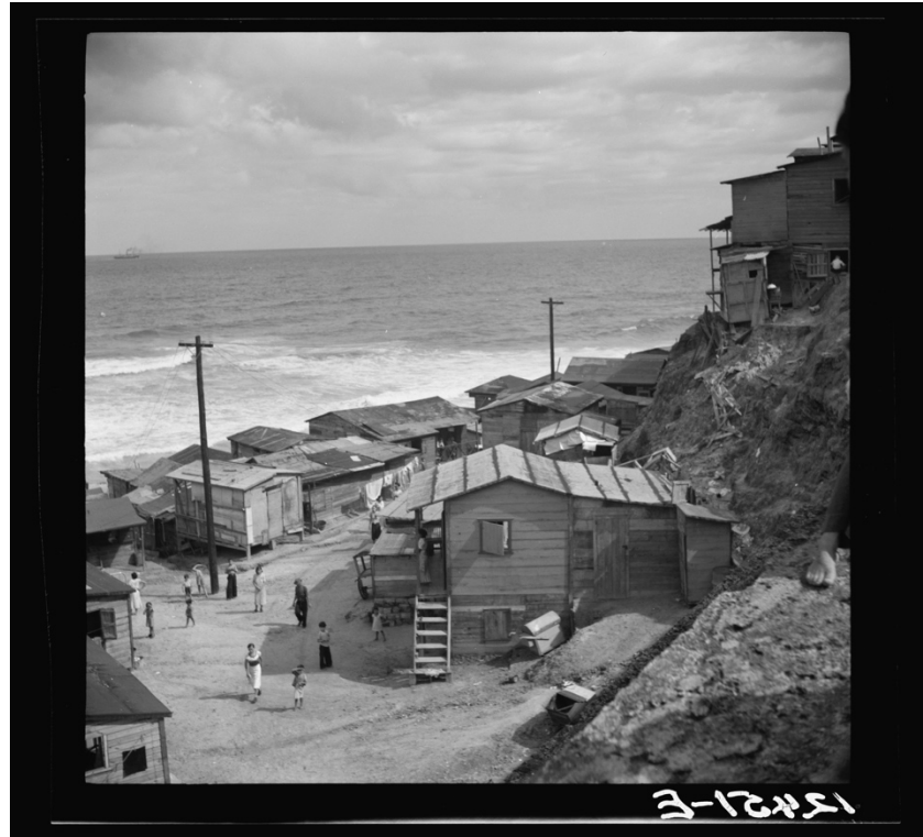
Figure 5: View of a portion of the workers' quarter of La Perla from the old Spanish ramparts, 1938, San Juan, Puerto Rico. Photo by Edwin Rosskam. Courtesy of Library of Congress, Prints & Photographs Division, Farm Security Administration/Office of War Information Black-and-White Negatives.
