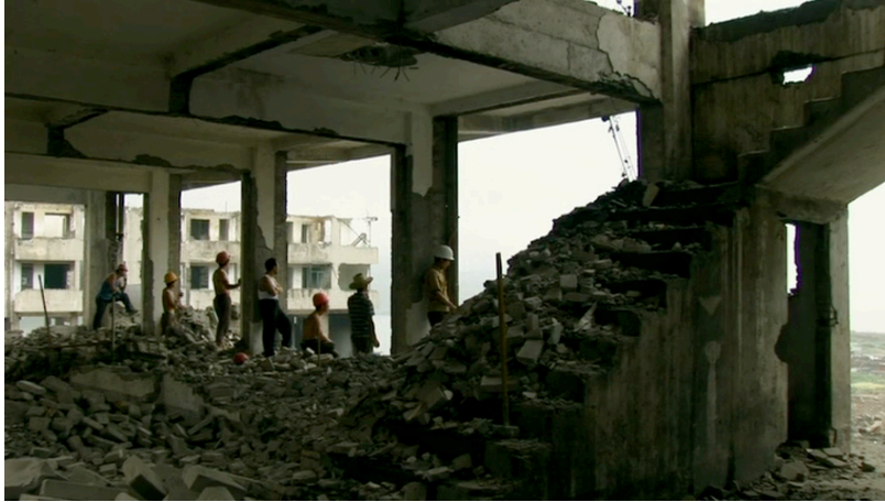
Figure 10 - Han Sanming and his demolition crew before they discover Mage's body
