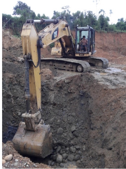
Figure 6. Excavator operator in Huepetehue. Photo credit: S. Antoni Delgado.
