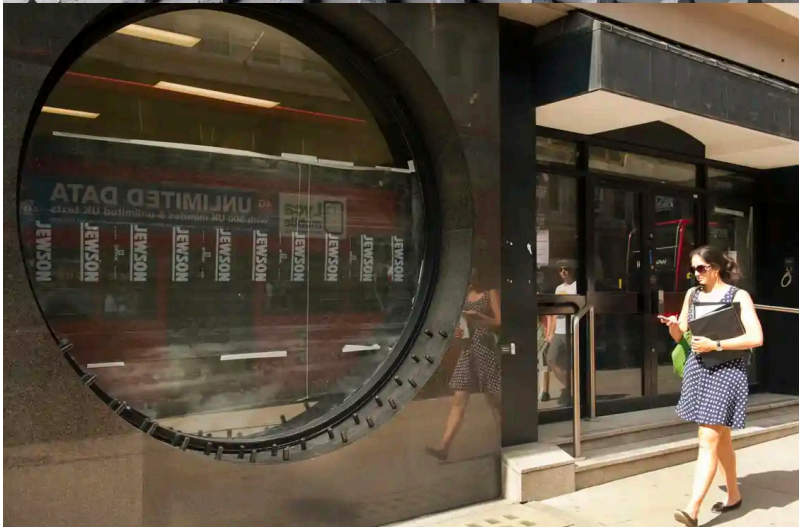
Spikes used to deter loitering in Coutts Bank, Fleet Street, London (Reed, 2015)
