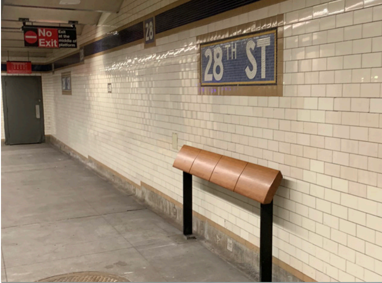
A leaning bench at the 28th street subway station in New York City (Kim, 2019).
