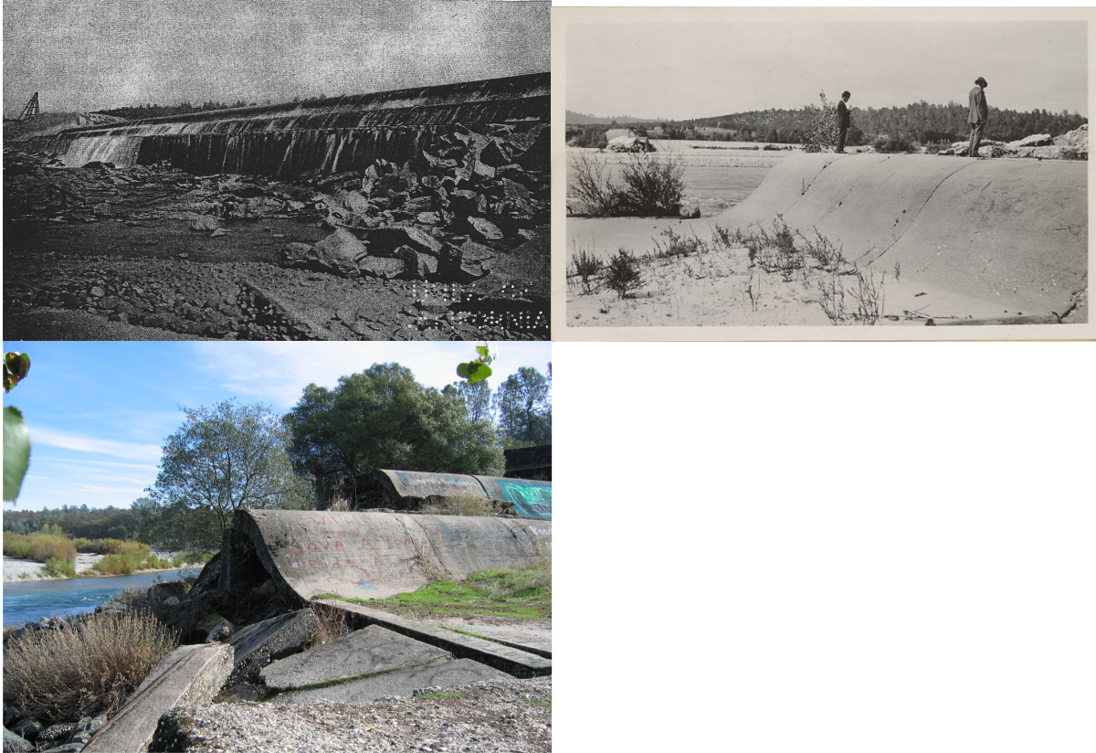
Figure 3. Lower Yuba River. Top– historical photo of Barrier No. 1 on the Lower Yuba River taken in September 1906 by Gilbert, just after completion and the season before it failed (Gilbert 1917). The debris dam was built by the California Debris Commission in 1904-1906 and was breached by floods on the Yuba River in 1907 (Gilbert 1917). Middle - historical photograph of Barrier No. 1 by Lippincott in 1913, six years after the dam failed (in University of California, Water Resources Center Archives, Lippincott collection). Bottom – the remains of the same dam in 2006 (photo by J.T.Minear). The bed of the river is approximately 7 meters lower than the base of the dam.
