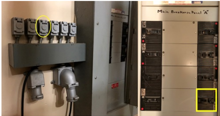
Figure A.5: Electrical Plug and Breaker for NR1500ZAG Rotation Table
