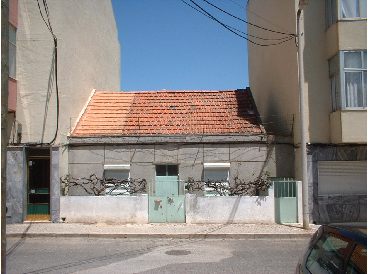
Figure I.7. Brandoa in 2009: Pre-1965 house on Almeida Garrett Street, in the Brandoa ward of the suburban Amadora municipality.
