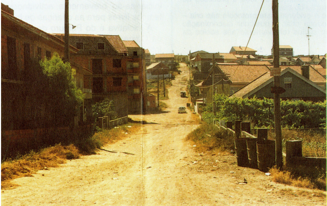
Figure 3.8. Casal de Cambra before the paving of the streets in the early 1990s. Note the concrete structure and brick infill of the unfinished buildings to the left, and the variation in setbacks of the open-lot structures. Note also the lack of parked automobiles at this moment in the history of the subdivision. Unknown author. Photograph courtesy of the archive of the Junta de Freguesia de Casal de Cambra (i.e. Ward Administration of Casal de Cambra, hereafter referred to as JFCC).
