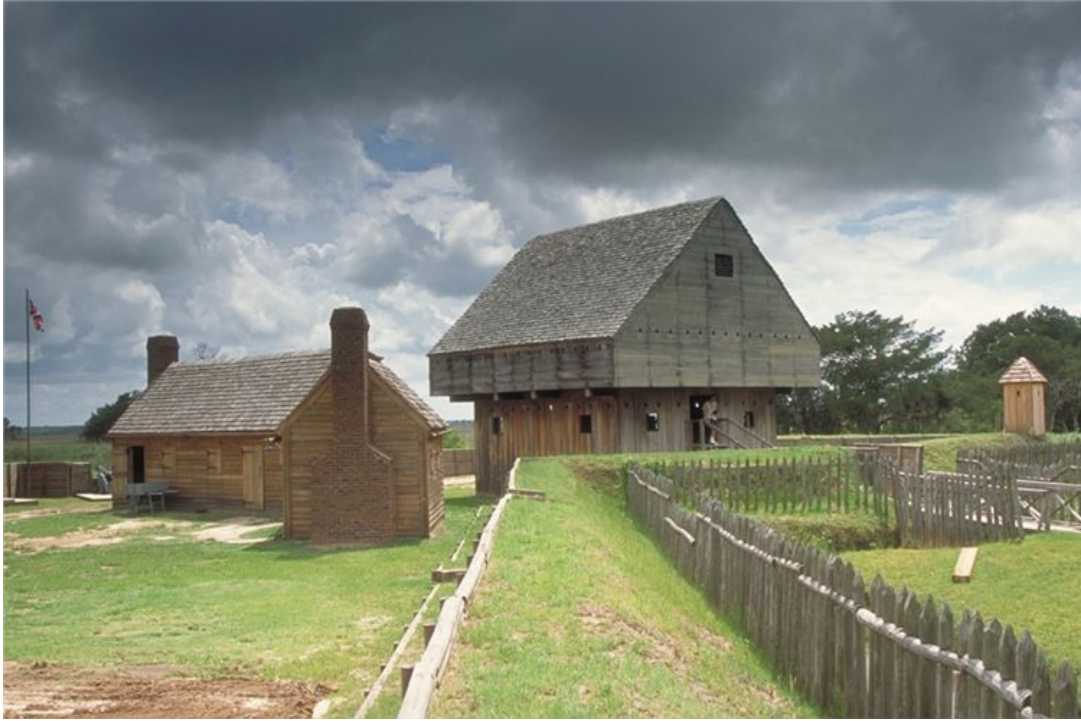
Figure 6.3— Current Reconstruction of Fort King George 17
