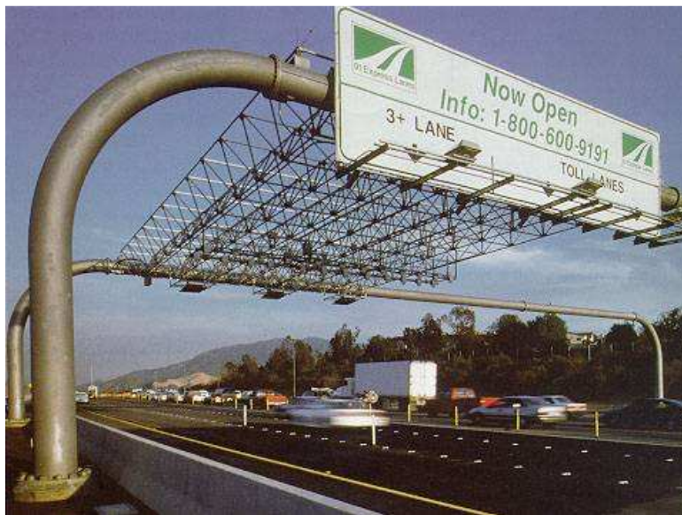
Figure 13 Self-Declaration Lanes for the SR-91 Express Lanes in Orange County 10
