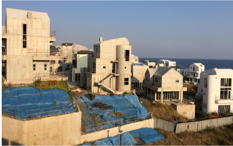
Figure 24: Unfinished Airst City complex. 233
