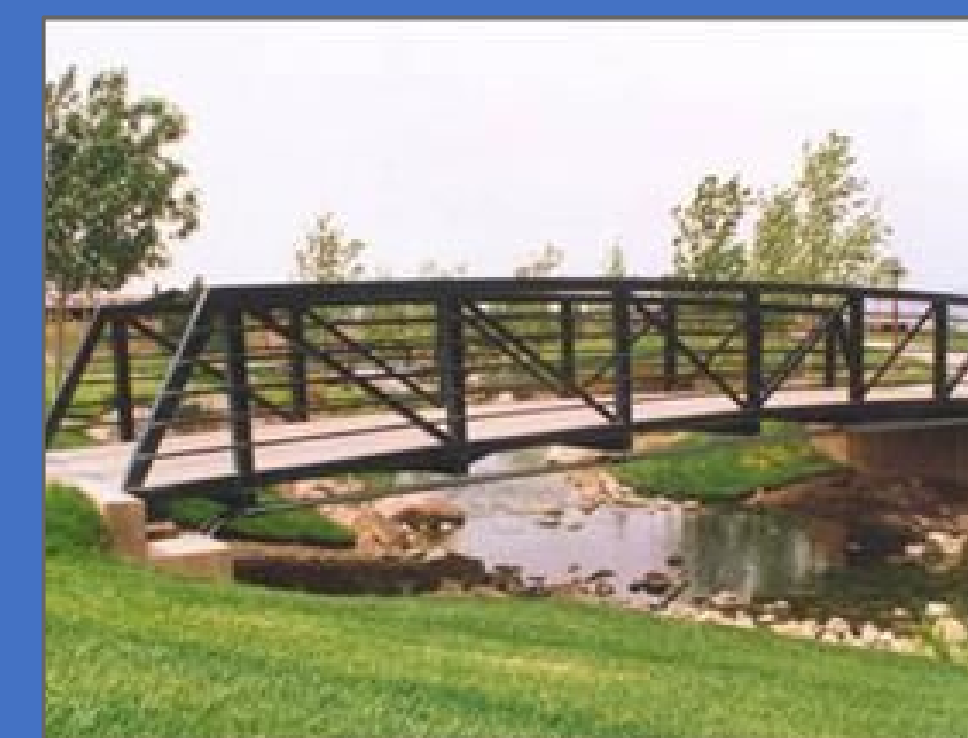
Continental Truss Bridge
