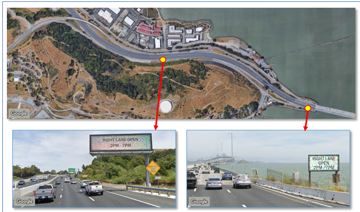
Figure 2-15: Dynamic Sign Indicating Shoulder Lane Open Status
