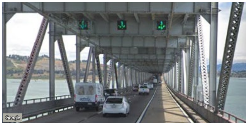
Figure 2-13: Electronic Lane Control Signs on Lower Deck
