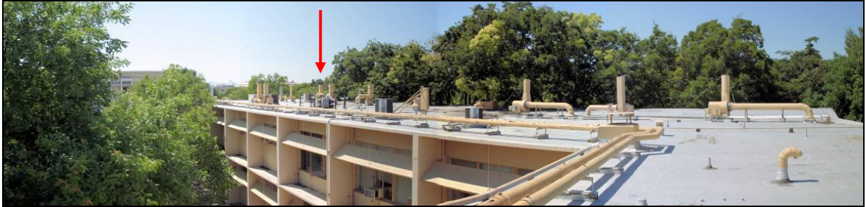
b) View from east edge of the roof.
