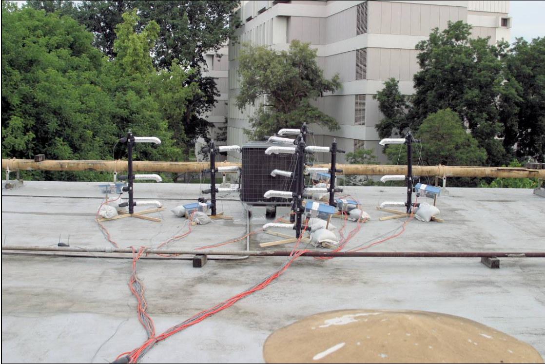
Figure 6. Views of the aspirated air temperature towers surrounding the test RTU. The plastic box attached near the bottom of each tower contains the aspirator fan and discharges downward. Sandbags were used on the tower bases to prevent wind from moving the towers.
