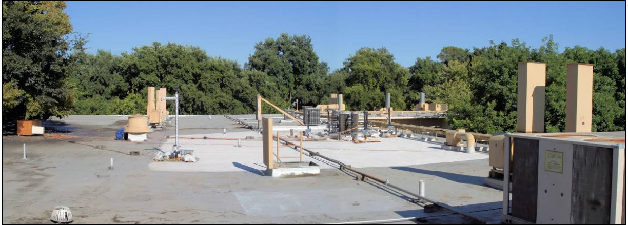
b) View from northwest.
