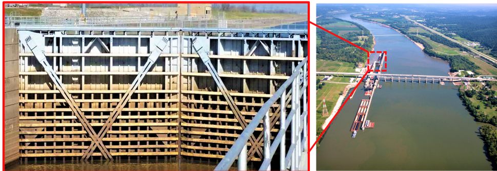
Figure 1: Greenup locks and miter gate
