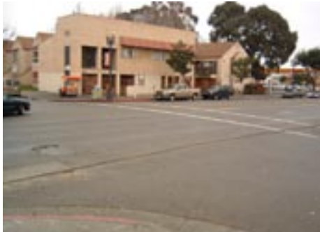
Looking southeast with view of southerly crosswalk
