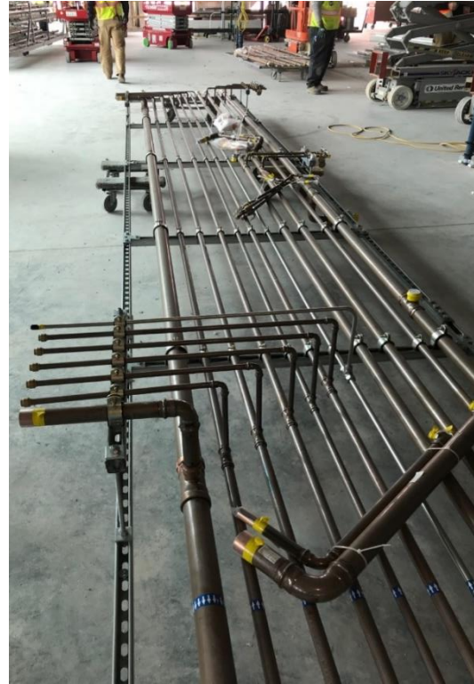
Figure 16: Prefabricated Pipe Rack
